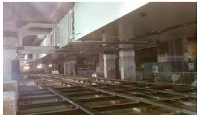
The next stage of this epic build was to fit the "vierendeel" girders, also constructed at ASG, into the roof which the spine would eventually be fixed to, but with the floor proving to be too weak to lift from, all structures would have to be hoisted from the concrete slab above.
