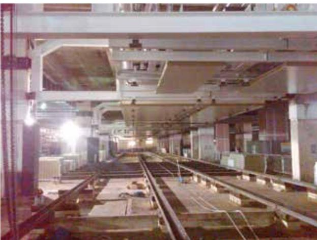
Working nights to avoid disruption to the station and other trades, a team of up to 8 operatives would then take delivery of the spine modules, 2 at a time, craning them onto the purpose built track and bolting the 2 spine modules together to create 1 section before beginning the task of pulling the section the full length of the station with a specially designed “tirfor” pulling tool.
