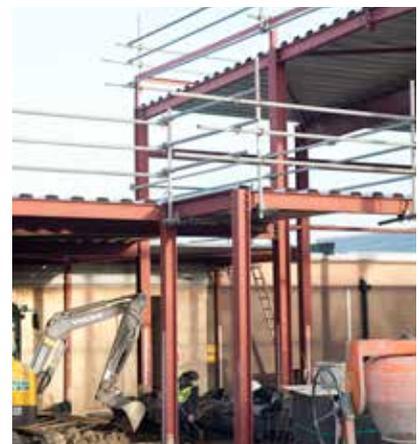
New assembly hall with link corridor and re-modeled dining area. ASG undertook the design, supply and installation of the main structural steel frame and internal steelwork alterations.
