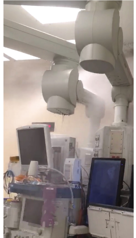
Figure 2: This figure depicts the water pouring down over the top of the machine after spraying out of the sprinkler system above.
