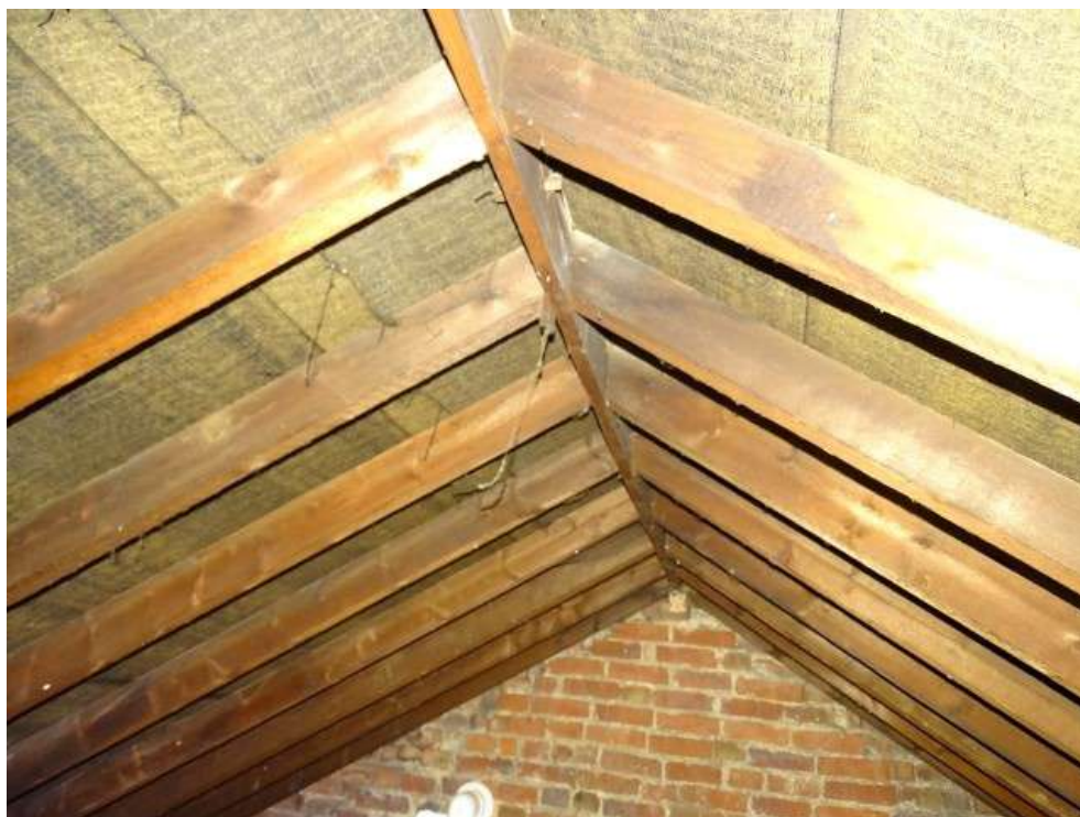
General view of roof structure
