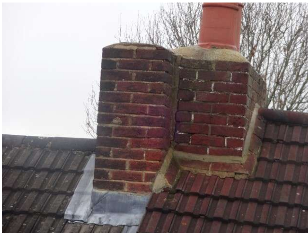
Main chimney stack
