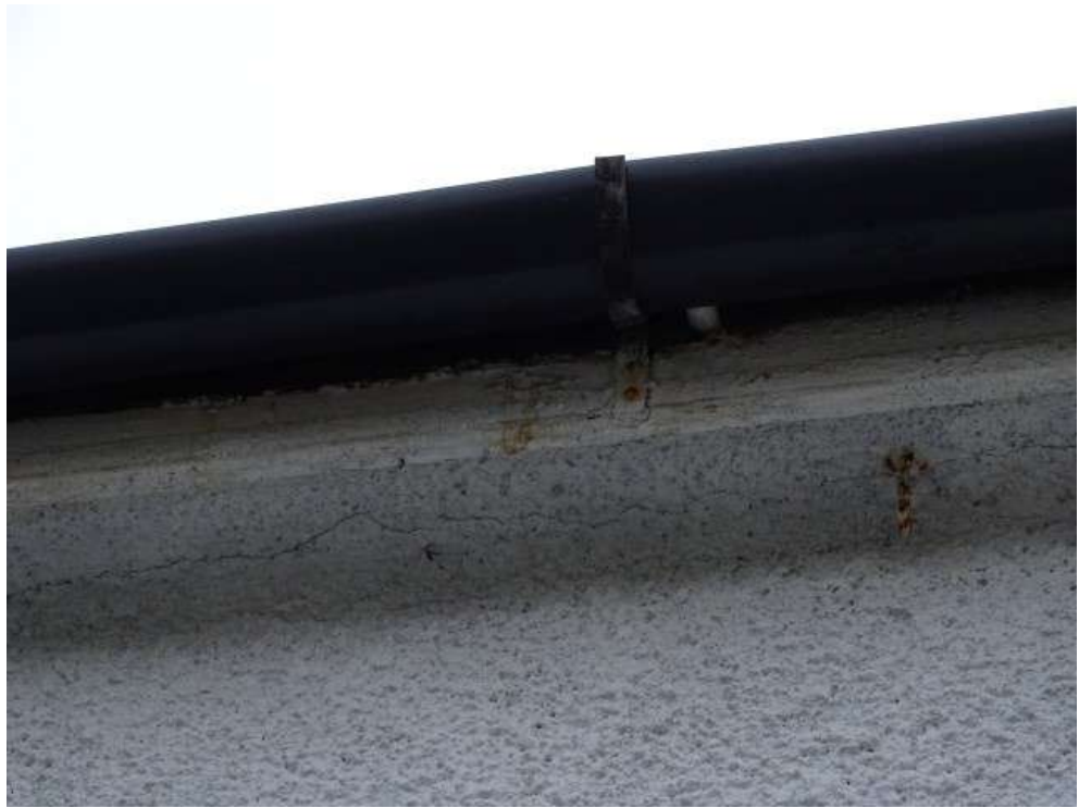
Rear gutter to main house
