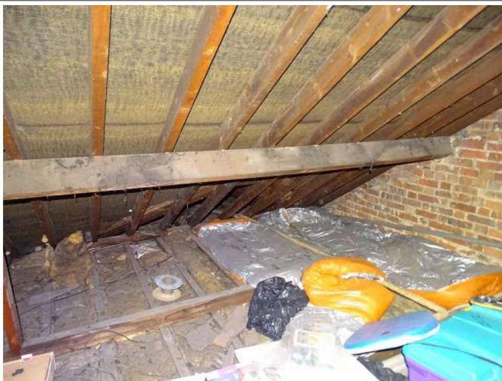
General view of roof structure
