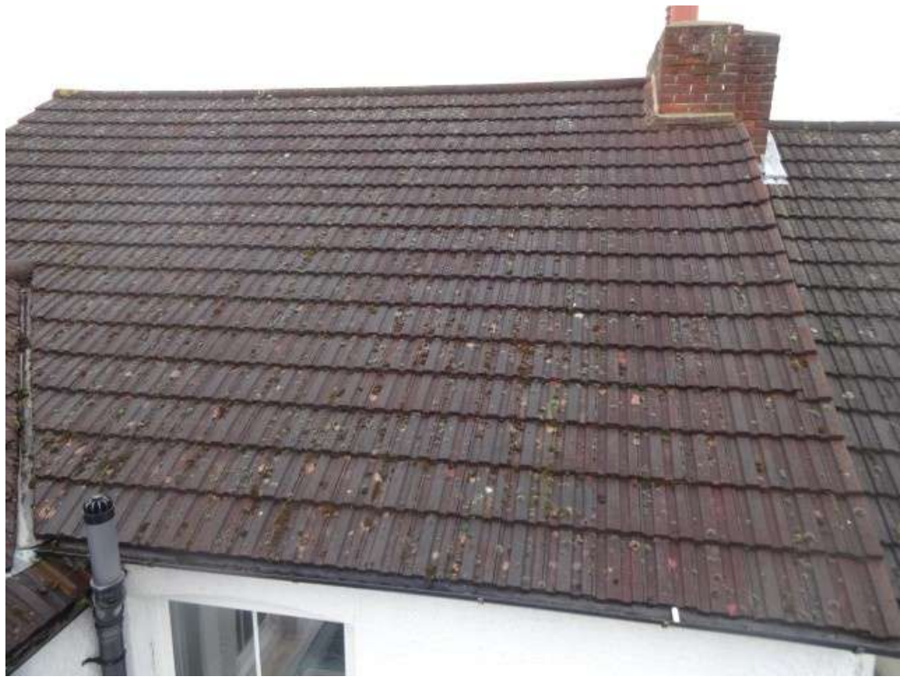
View of rear roof slopes using pole camera
