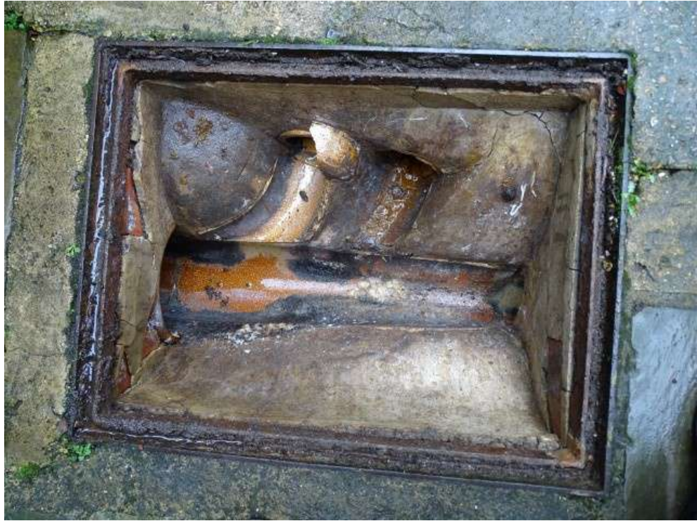
Main drain in alleyway
