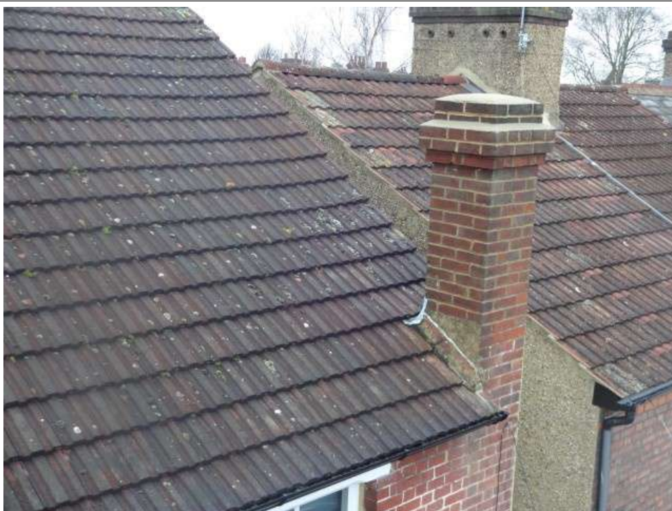
Front bedroom chimney stack
