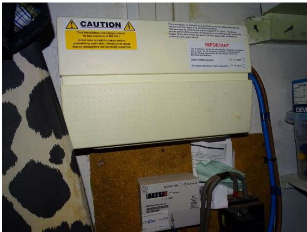
Electric meter and consumer unit
