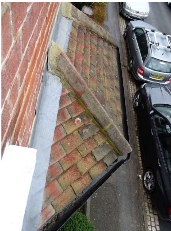
Roof to sitting room porch roof
