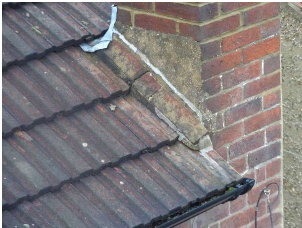
Tiled flashing to chimney stack
