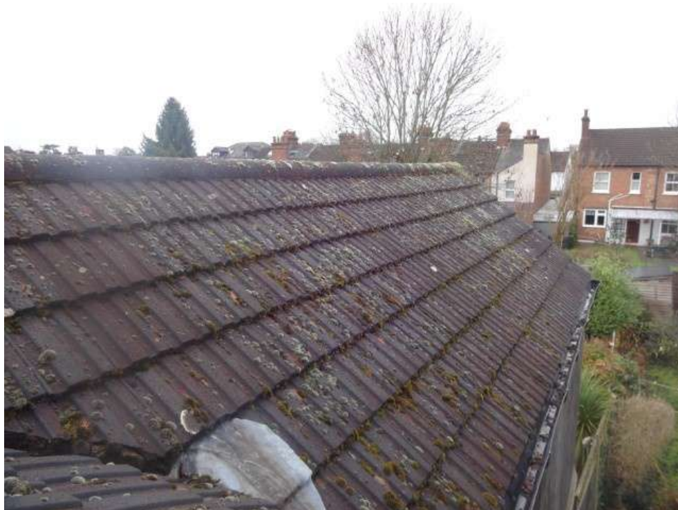
Rear roof over Bedroom 4
