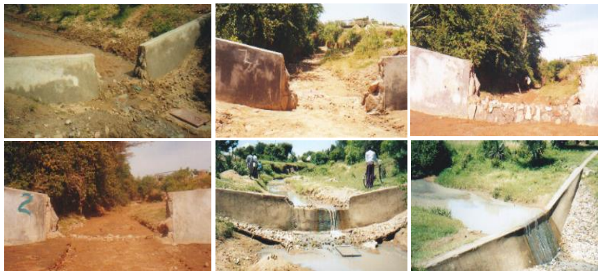
Figure 2: A sand storage dam was raised 3m in 6 stages of 0.50 m in one rainy season, in Kenya. Source: (Nissen-Petersen, 2006).
