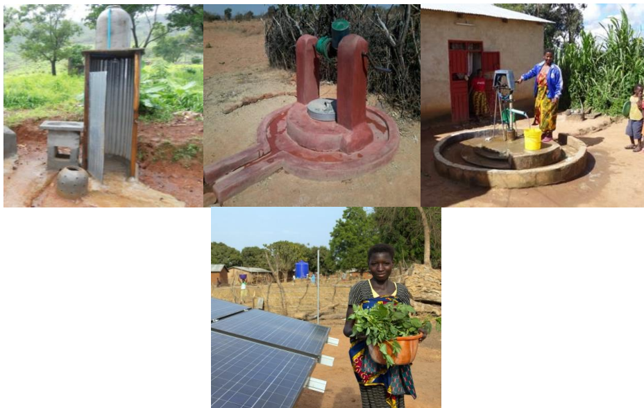
From left to right: EMAS overhead tank for shower; upgraded family well; rope pump working for 6 years; solar pump for multiple use of water
