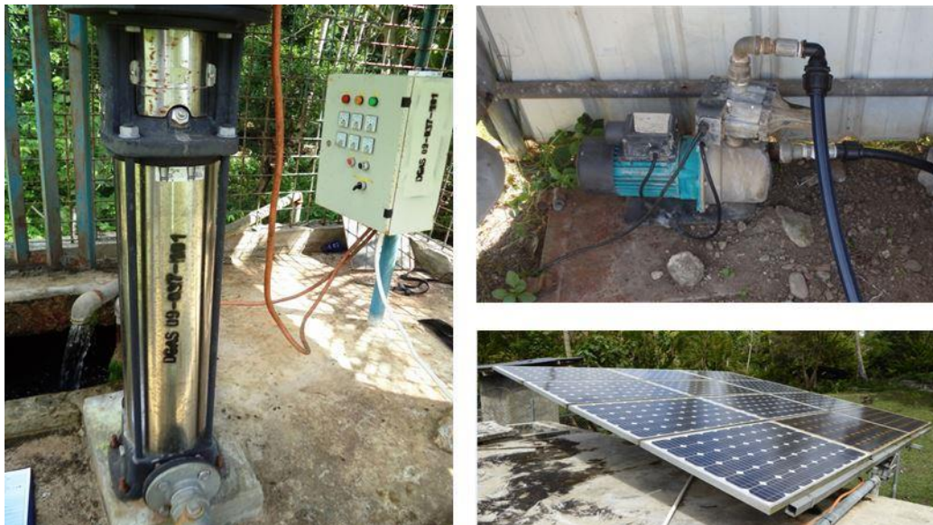
Figure 3-42: Types of pumped water systems in rural areas, large centrifugal pump (left), small centrifugal pump (top right) and solar submersible pump (bottom right) (BESIK, 2015b)
