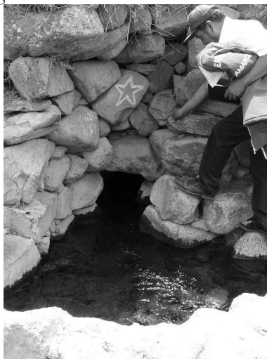
Fig 14. - Andamarca spring had a flow rate in excess of 40 l/s
