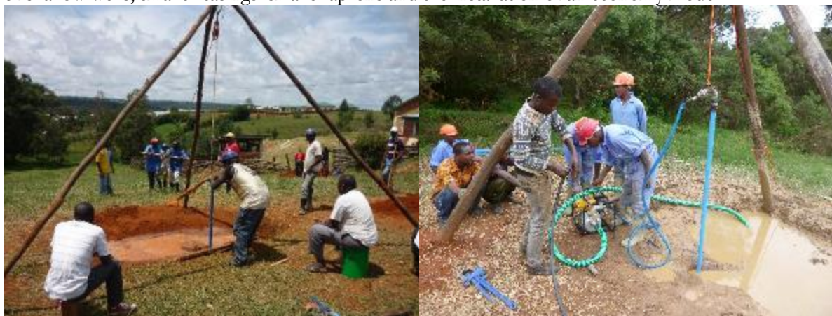
Drilling a tube well of 30 meters deep with the SHIPO drill method The SHIPO drill combined with jetting
