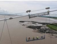
requirements' ALPS designed an access system that used the hand strand cables as primary support, this leaving clear & unloaded the main bridge suspension cable for wrapping works.
