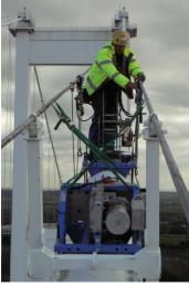
The Severn Bridge engineers required a simple & effective access method enabling them to carry out main cable wrapping during initial cable dehumidifying works. After consultation with the bridges engineers' and establishing the actual project
