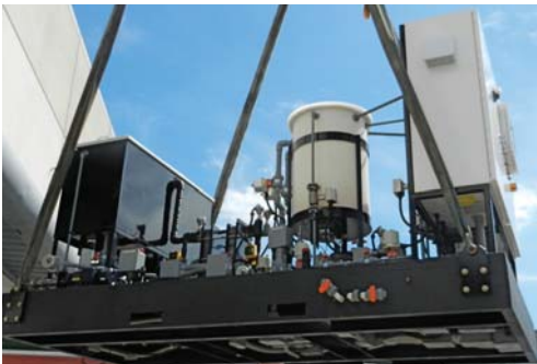
Hoisting an Fe70 Ferrator for New Orleans
