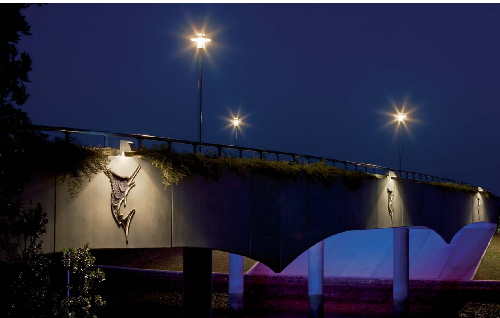
Endeavour Bridge, Whitianga Waterways. Whitianga (NZ). Lighting design: Airey Consultants / Modus Lighting.
