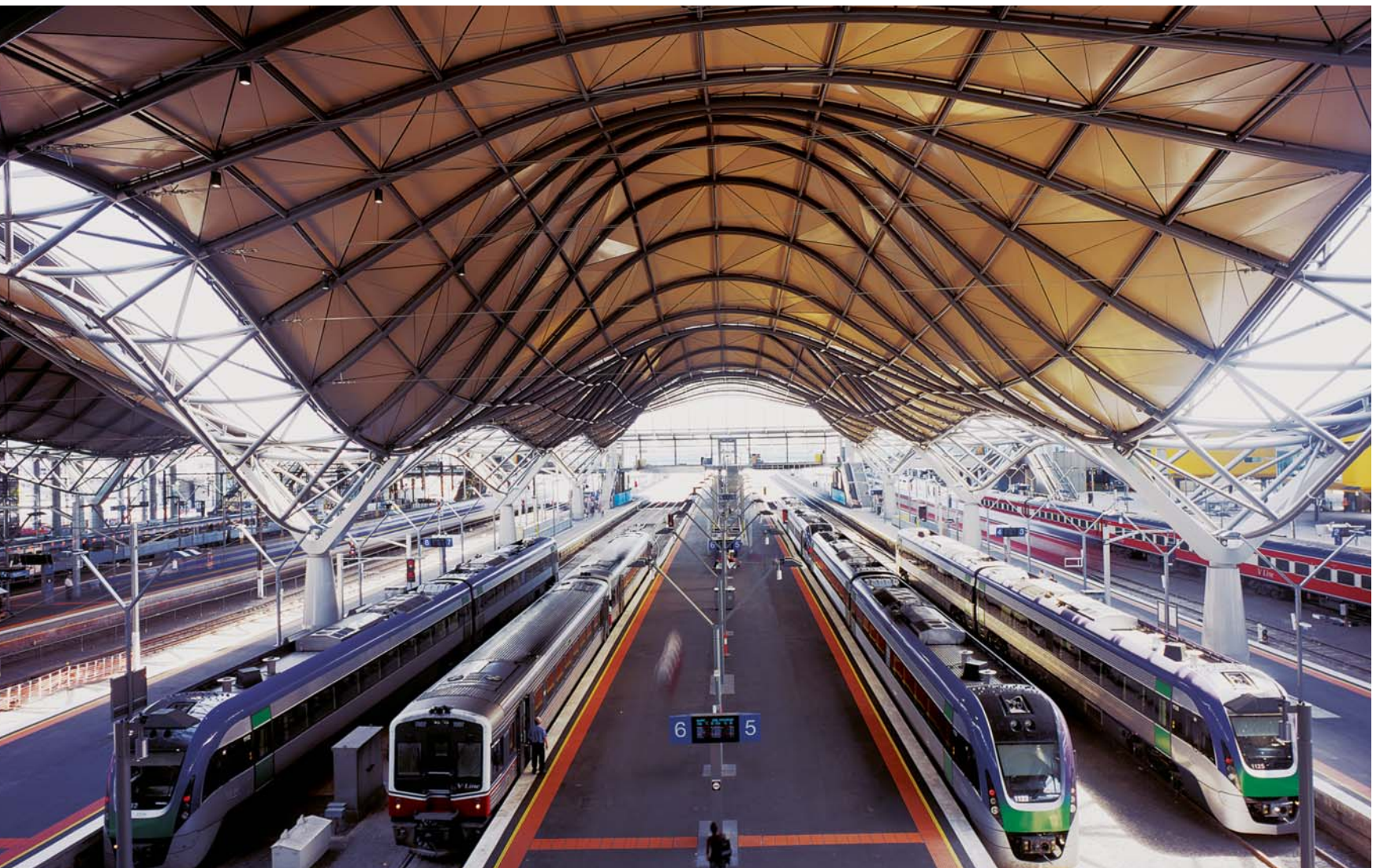
Southern Cross Station. Melbourne (AUS). Architect: Nicholas Grimshaw & Partners. Lighting design: Vision Design Studio.
