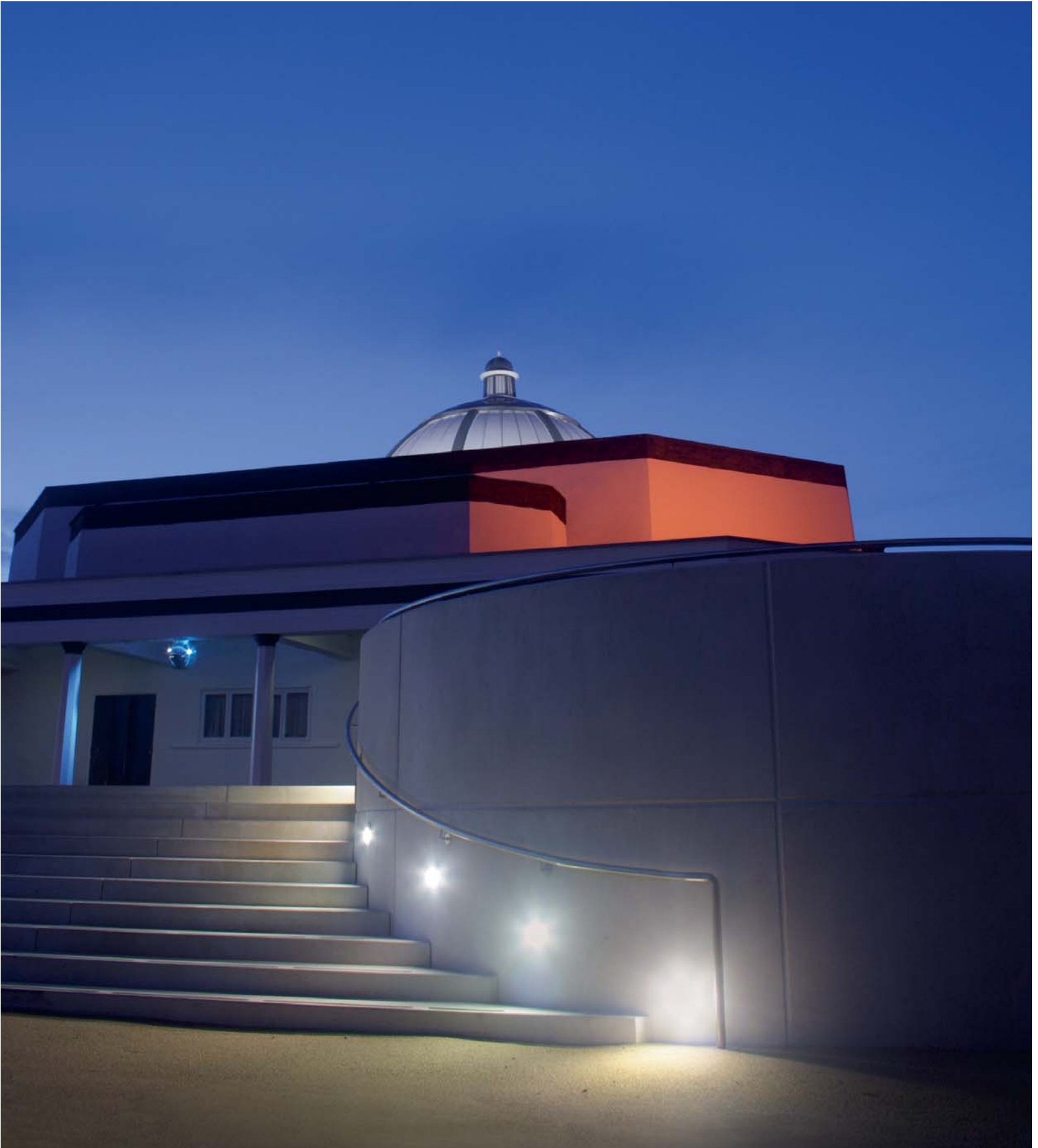
Marine Hall Gardens. Fleetwood (UK). Landscape architect & Lighting designer: BCA Landscape.
