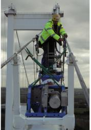
The Severn Bridge engineers required a simple and effective access method to enable them to carry out main cable wrapping during initial cable dehumidifying works.
