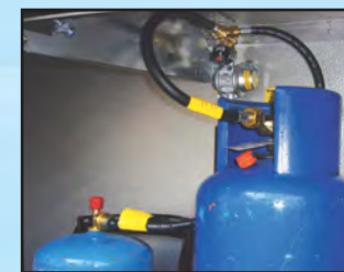
A twin system with a 0.45m and 0.75m rubber hose using a Gaslow Manual Changeover Adapter (01-1626) connecting a Camping Gas and a 7kg Butane cylinder.
