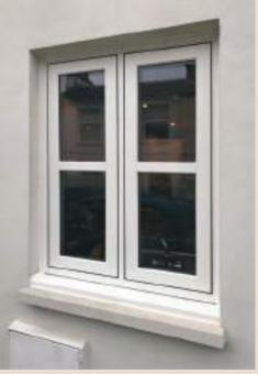
The above two photos show Ultimate Heritage flush windows in both vertical and horizontal opening styles, both with dummy sashes in the fixed windows to maintain balanced sightlines.
