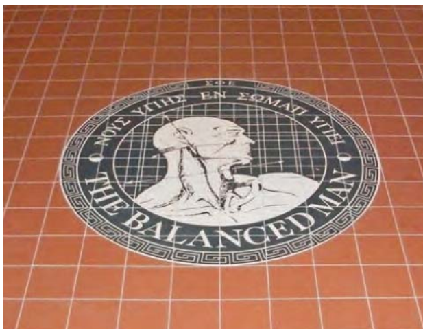
Logo printed black on white tiles then cut by water jet for precision. Tiled into a field of red 151mm/6" squares. From sketch to finished foyer.
