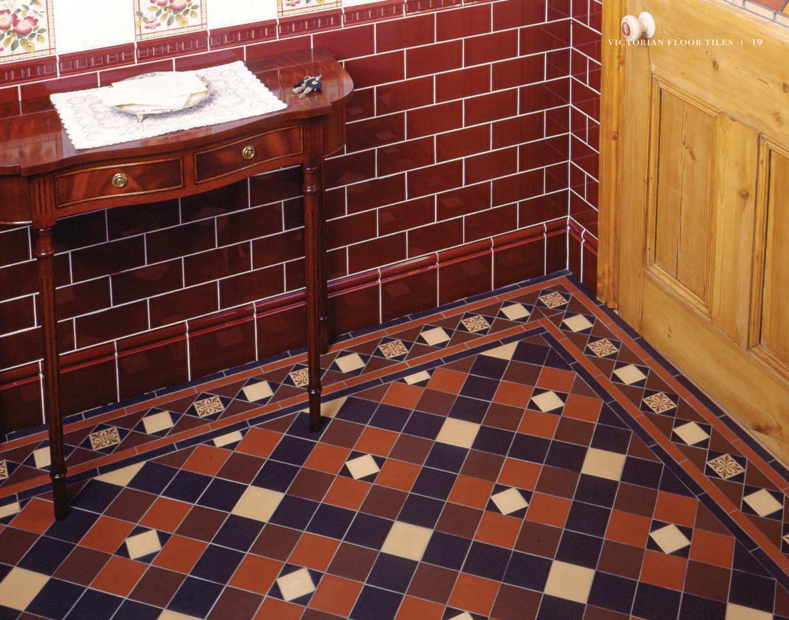
▲ Richmond pattern in Red, Brown, Buff and Black with modified Browning border incorporating Cardigan Brown on Buff decorated tiles. Wall: Original Style Artworks Half tiles, Skirting and Dentil moulding, all in Burgundy
