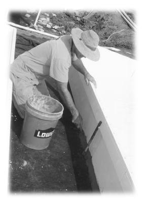
Sealing slant troughs to the Mirafi geotextile ground cloth with mortar and a trowel keeps mice, bugs, and dirt out from under your troughs.
