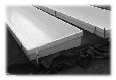
"Slant" troughs in a "sloped" grading installation. Note airlines with valves stubbed-out, pipes in VERY shallow trench to left (rocky ground!), Mirafi ground cloth ready to finish installation after trench is backfilled.
