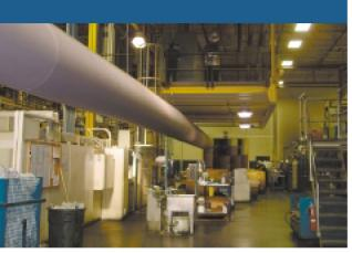
type of DuctSox, the Low-Throw Sedona model, which was custom manufactured with a porosity that allows all of the air to flow through the fabric within Fina's airflow velocity requirements of 15 ft./second. The winter DuctSox, which use the same H-track cable suspension system as the summer DuctSox, distribute 100-percent outside air that's tempered to 55°F to 65°F. The even and gentle air dispersion through the material allows the building's air to stratify, with the cooler fresh air near the
