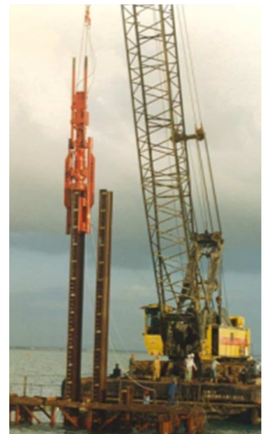
Figure 21 Mouton Diesel. Source : Delmag.com →
