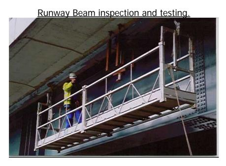
A 6M X 800mm alloy suspended access platform is installed to the new runway beams. The beams and fasteners are examined and proof load tested using the special calibrated jacking system designed by ALPS for this application. The test load can be held in place whilst the fixings are examined.
