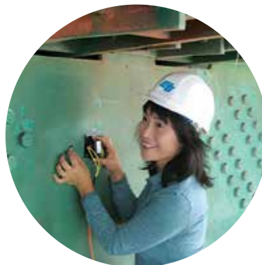
Testing new sensors at the Vincent Thomas Bridge, a 1,500-foot-long suspension bridge in Southern California
