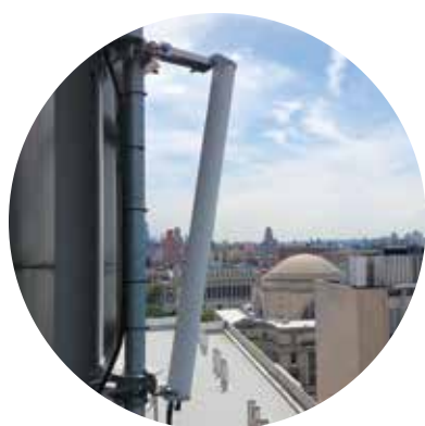
A WiMAX base station (on top of the Mudd Building) used for hands-on experimentation in Electrical Engineering and Computer Science networking classes.
