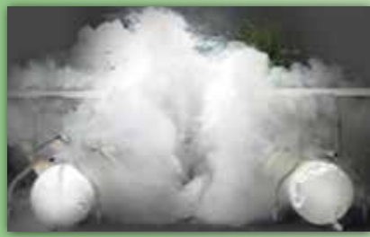
Slow air dispersion through the fabric results in uniform airflow.
