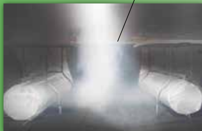
High velocity discharge causes localized drafts.
