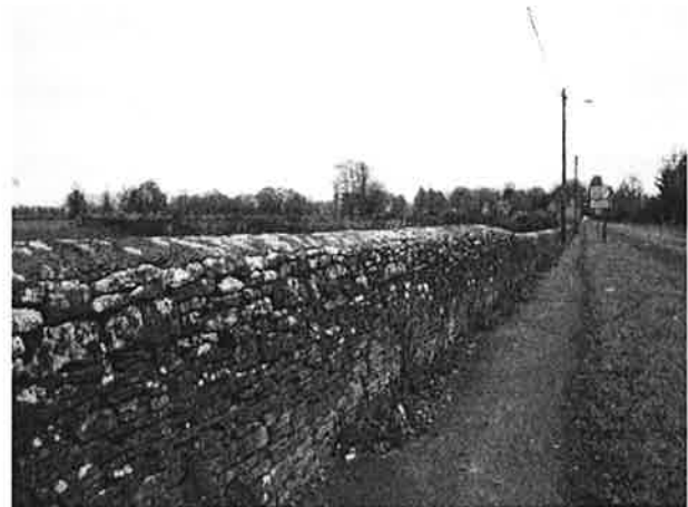
Figure 3 - Site Access B would result in the loss of 80 linear metres of drystone walling.
