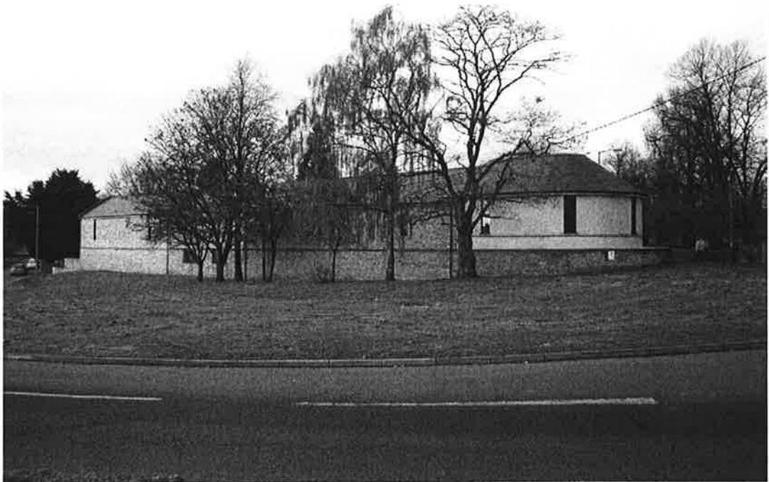
Figure 10 – Commercial property at Pickwick Park directly to the south of the proposals has been sympathetically designed on the boundary of the Pickwick Conservation Area and contributes to the settlement gateway of north Corsham. The proposals would detract from the settlement gateway.
