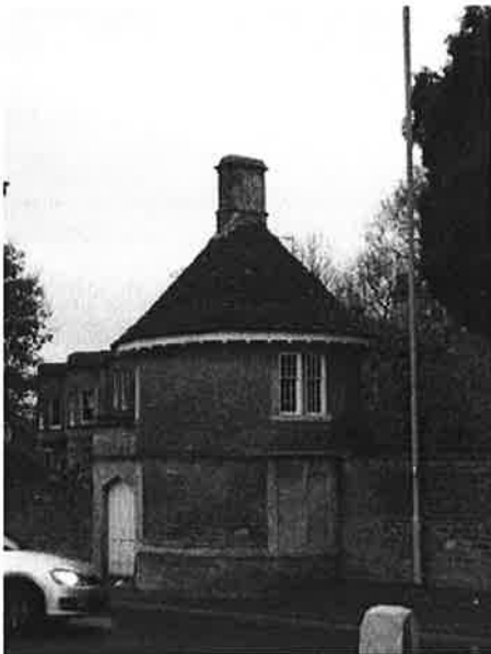
Figure 12 – the setting of the Roundhouse that marks the settlement gateway into Pickwick would be compromised through extended built form to the north of the A4. Tollhouses were historically at the entrance to a settlement and this perception would be lost as a result of these proposals.
