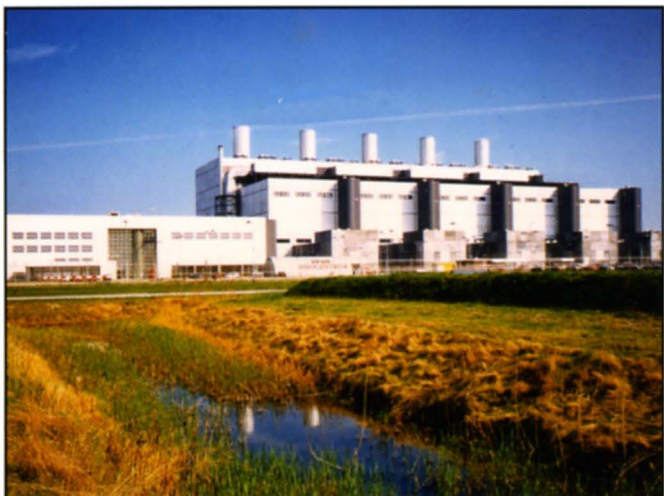
Electrabel Nederland BV, Netherlands Eemscentrale, General Electric Frame 9FA
