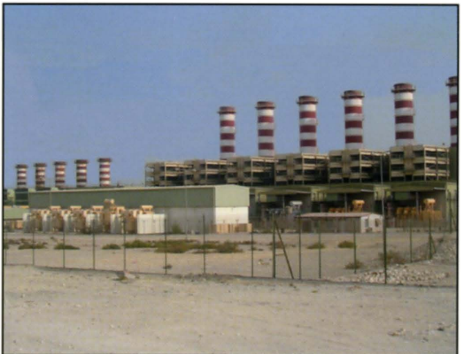
Ministry of Electricity and Water, Bahrain Rifaa, Siemens Model V93.1 and Alstom GT13D
