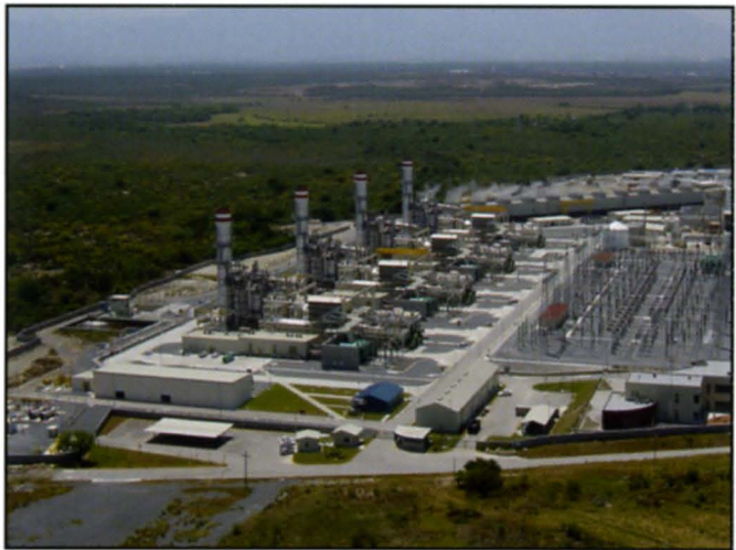
Iberdrola International and CFE, Mexico Monterrey, Alstom Power GT24
