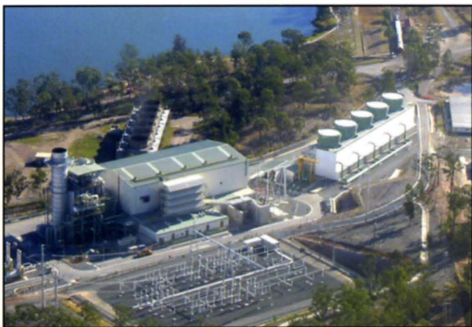
CS Energy Limited, Queensland, Australia Swanbank E, Alstom Power GT 26
