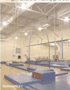
Hammelman began designing the main gym's air distribution around the standard of six volumetric air changes per hour which typically allows for a 10-degree breakpoint for non-cooling situations.
