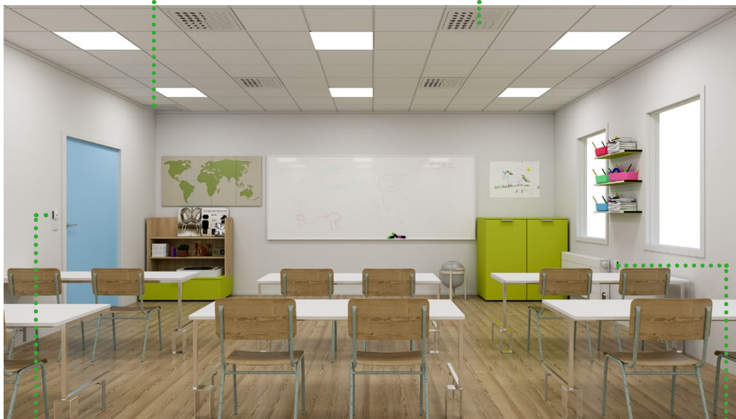
Passive supply air diffuser
