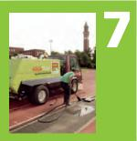
Aquatrax® can also effectively clean trackside drainage systems. As only water is used, the waste can be discharged in to a foul drain.
