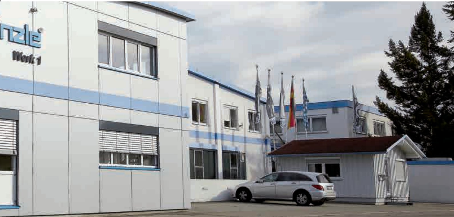
Production factory 1, Illertissen
