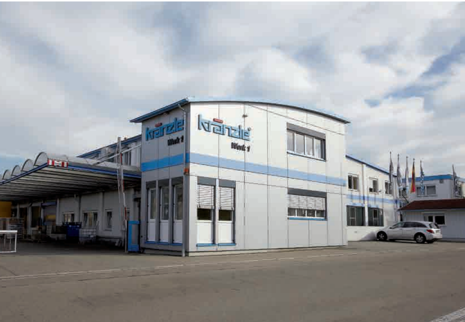
Production factory 1, Illertissen
