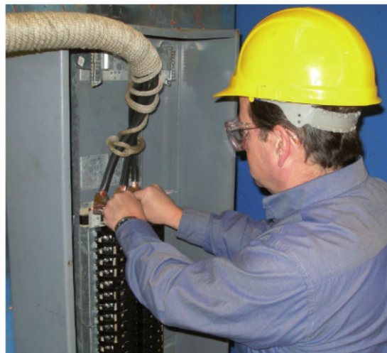
Setting up an arc flash test on actual equipment - NEMA (U.S.) panelboard
