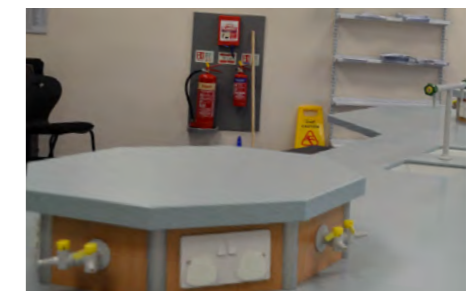
Many shapes of service turrets are available and can incorporate Power, Data, USB & Gas.
