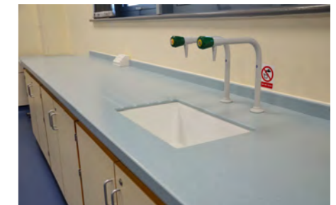
Under mounted sinks with machined draining zone.
