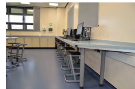
Perimeter knee space can be provided with or without support legs depending on wall strength.
