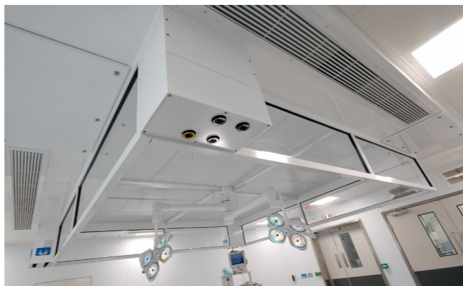
Laminar flow canopy with 3.5m 2 clean zone
