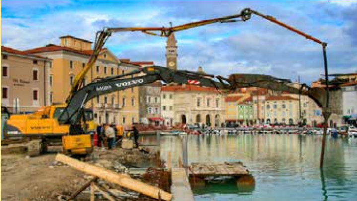
Underwater concreting - Arm extension enables concreting in a higher water depths (longer distance). It guides the funnel to required depth and enables underwater concreting. Working (digging) with Long Reach Arm enables reaching the larger digging distances, overcoming some physical obstacles and reach positions that are much above or below the excavator level, which increases working efficiency.
