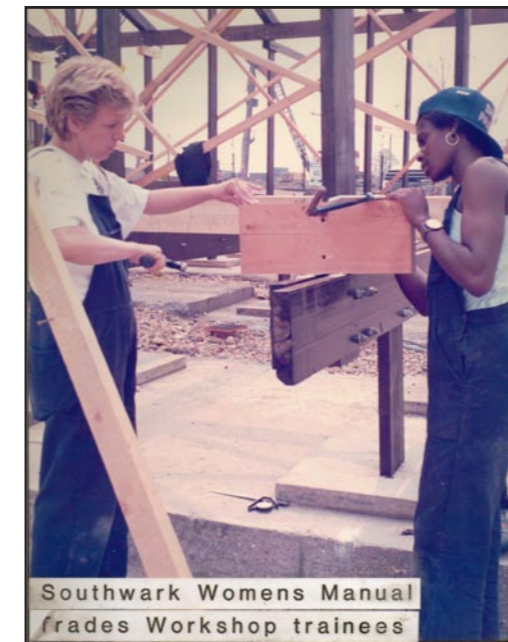
Above: trainees working on the construction of the Segal building.
