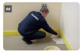
Working from the manifold location, start by laying end return and or transitional panels along one wall **(6g)** (working in conjunction with pipe layout drawing) **(6f)**.
