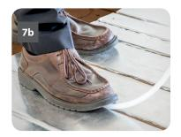
Walk the pipe into the channels in the overfloor boards ensuring the pipe is pushed securely into the bottom of each channel (7b).
