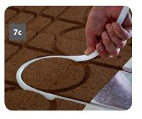
Pert/Al/Pert pipe: In the unlikely event of a kink in the pipe occurring, wrap the pipe in a cloth for protection and gently squeeze with pliers to re-shape
