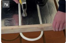
If pipes sit proud of the surface of the overfloor boards, make sure the channel below the pipe is clear from debris. The pipes can then be gently tapped down using a wooden batten laid across the board and pipe, then tapping with a hammer (7a).
