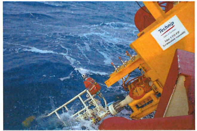
Figure 7. Installation of Islay ETH-PiP.
