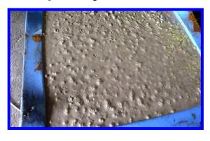
Correct vibration ensures the concrete is fully compacted and excess air is removed quickly and effectively.
