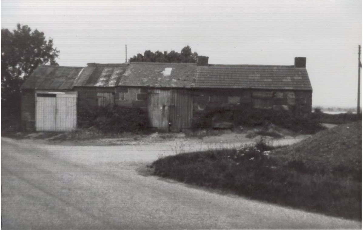
Fig 47 The building that was the blacksmith's shop
