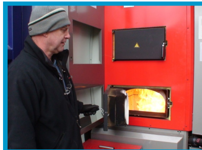
Commissioning the boiler
