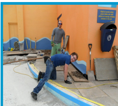
Volunteers Mike Thatcher and Nick Lewis relaying slabs surrounding the toddler pool
