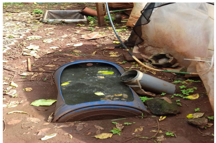
Bio-slurry ejected from the outlet of the biogas plant.
