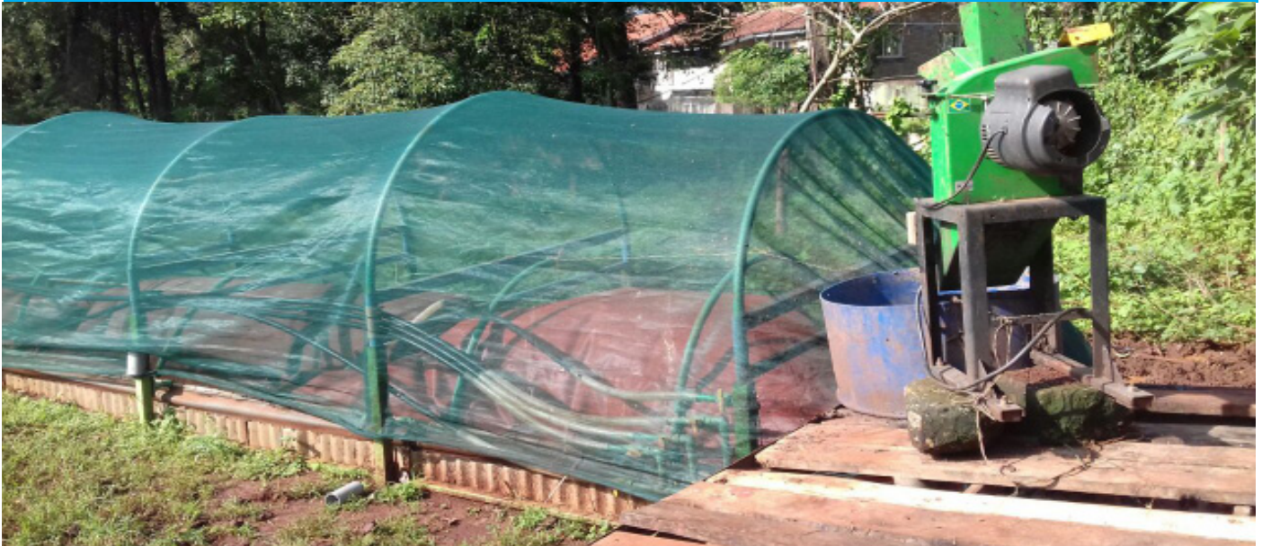
A commercial biogas plant at the eco-resource centre in Karen, Nairobi, Kenya.
