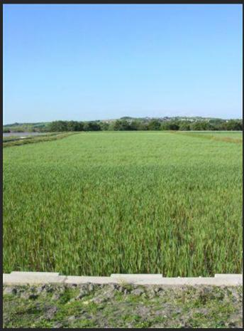
A 2.7ha reedbed for treating mine water discharge – design input, reed production, planting and initial maintenance were all undertaken by the consultants of AquaticEngineering
