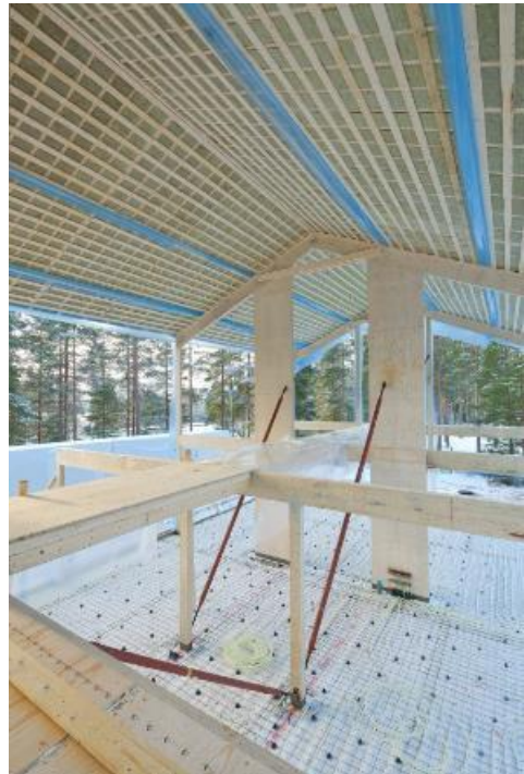
Post and beam
