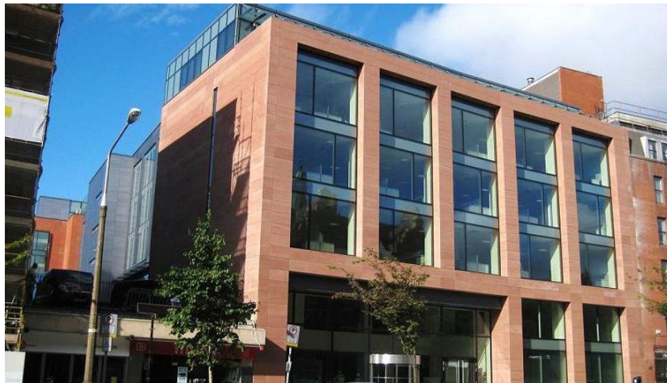
St Bees Cladding – Baggot Plaza, Baggot Street, Dublin
