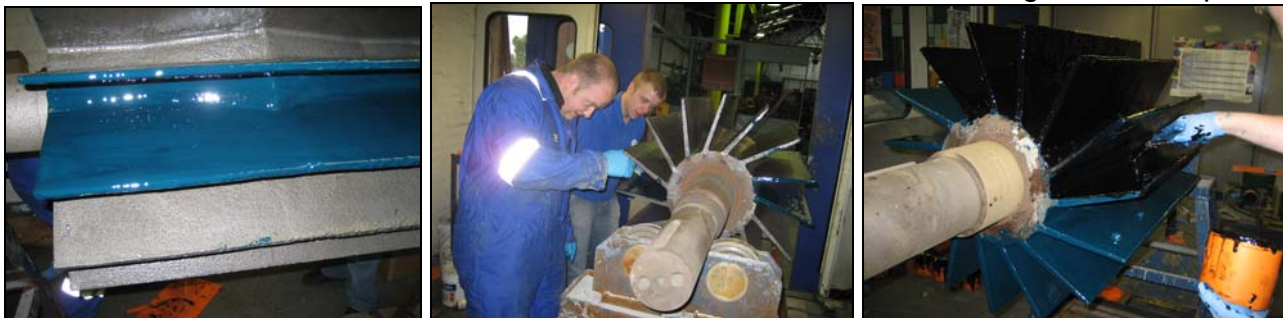
First coat of 214 - Impeller being coated - Applying second coat 2141
