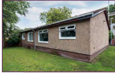
15 Finlaystone Place, Kilmacolm
