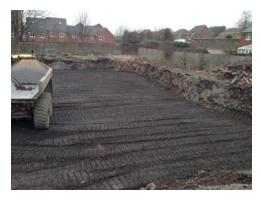
The soils treatment was contained within the concrete reservoir structure until the material was fully recovered, providing a secure treatment area. Initial reagent trials were undertaken with 4 day tank tests undertaken to assess the optimum reagent mix. Following Environment Agency deployment notification the soils were processed, incorporating much of the retained perched groundwater within the process.
