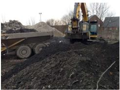
Stabilisation and solidification was chosen as the preferred treatment option to meet agreed leachate target criteria with the secondary benefits of preventing the need for hazardous landfill disposal, geotechnical improvements to the soils and the encapsulation of the residual asbestos risk.
