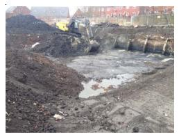
Our sister company Urban Regen Ltd was engaged by Morris Homes Ltd, to undertake full site preparation and remediation of the former mill site following discovery of a reservoir covering half of the development site post demolition by others. A subsequent round of investigation encountered heavy TPH contamination at the base of the reservoir, with geotechnically poor overburden.
