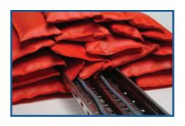
Passive fire protection is installed to maintain the integrity and structure of the building, this can be achieved by the installation of various materials to afford the fire rating required to create fire compartments throughout the building.
