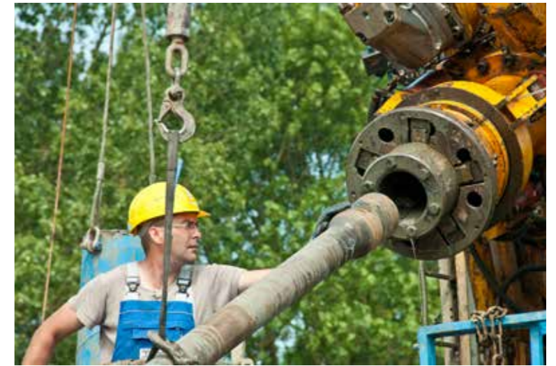
Installing drill pipe.
