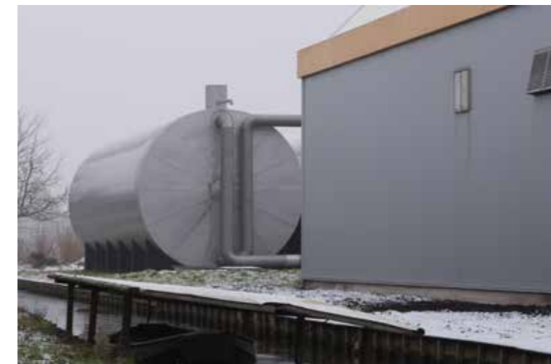
The large water buffer tank (400m³) allows the tropical plant nursery to benefit from lower electricity rates during off-peak hours.
