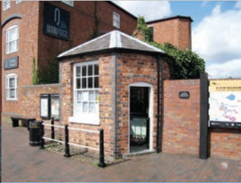
Above, the restored tollhouse at Farmer's Bridge Locks marks the start of the Birmingham & Fazeley Canal
