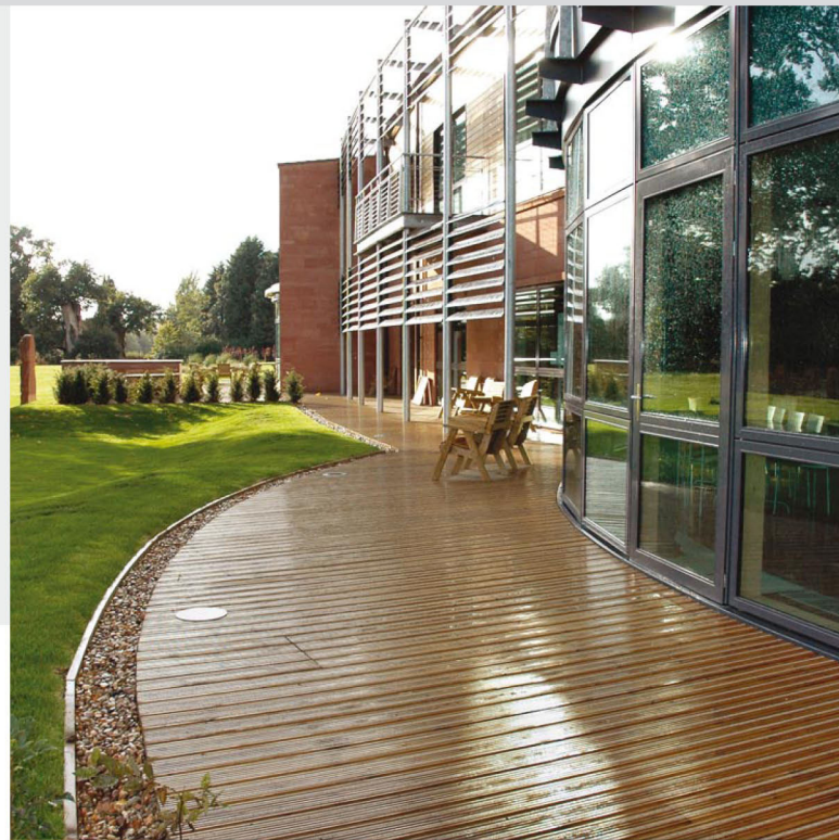
Ground level decking: John Brash & Co Ltd.
