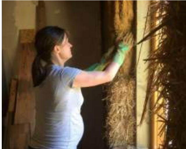
Erica Thompson applies locally-sourced plaster to the straw bale insulation in her new house. Thomas Reuters Foundation / Max Baring
