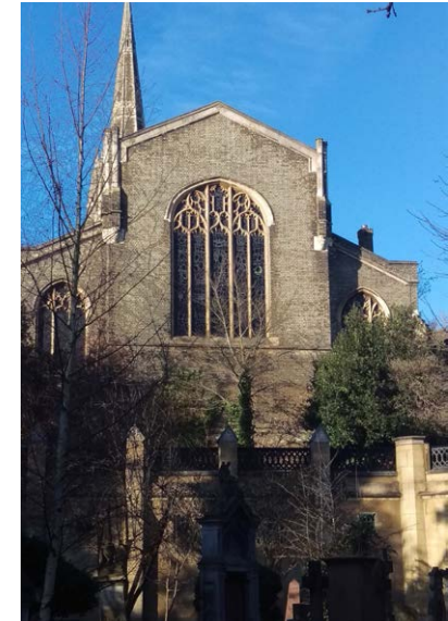
Fig 72. Tree clearance has opened up views of St Michael’s Church and the setting of the catacombs
