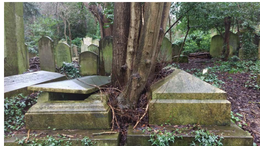
Fig 89. A multi-stemmed Elm growing between 2 tombs and causing damage in West Cemetery
