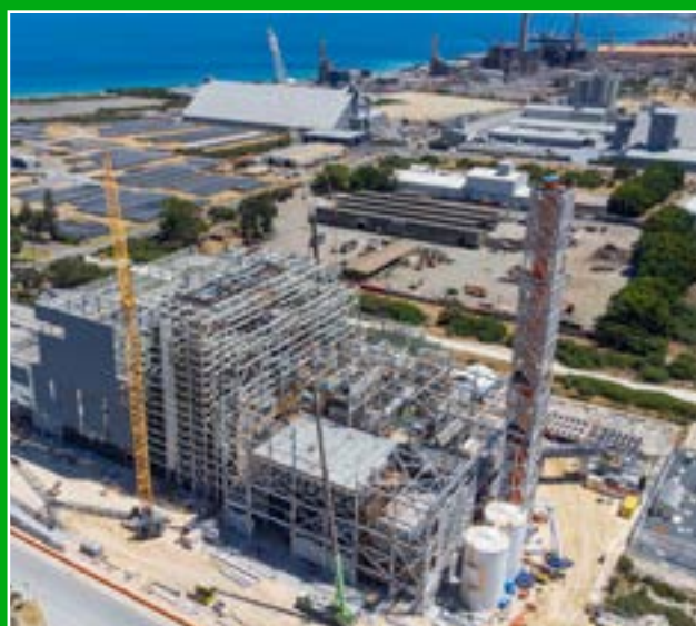
Avertas Energy Facility taking shape Cover image credit: Avertas Energy
