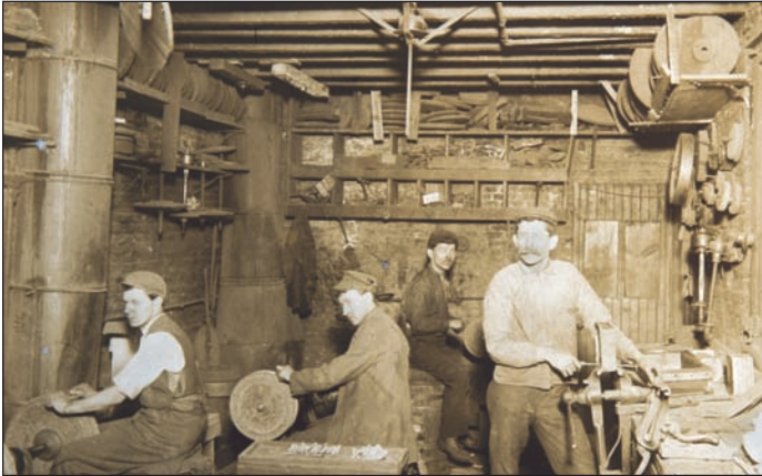
Workers putting the finishing touches using grinding wheels
