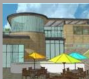
Boringdon Hall Hotel Page 3
