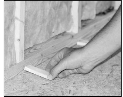
Figure 3.1: Place shims on floor in front of base plate
