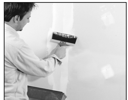
Figure 3.4: Tape and mud drywall
