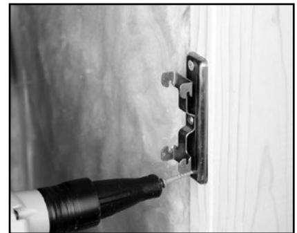
Figure 2.2: Secure second anchor
