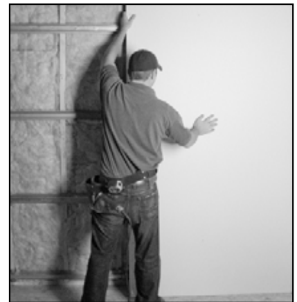
Figure 3.2: Install drywall vertically to hat channels
